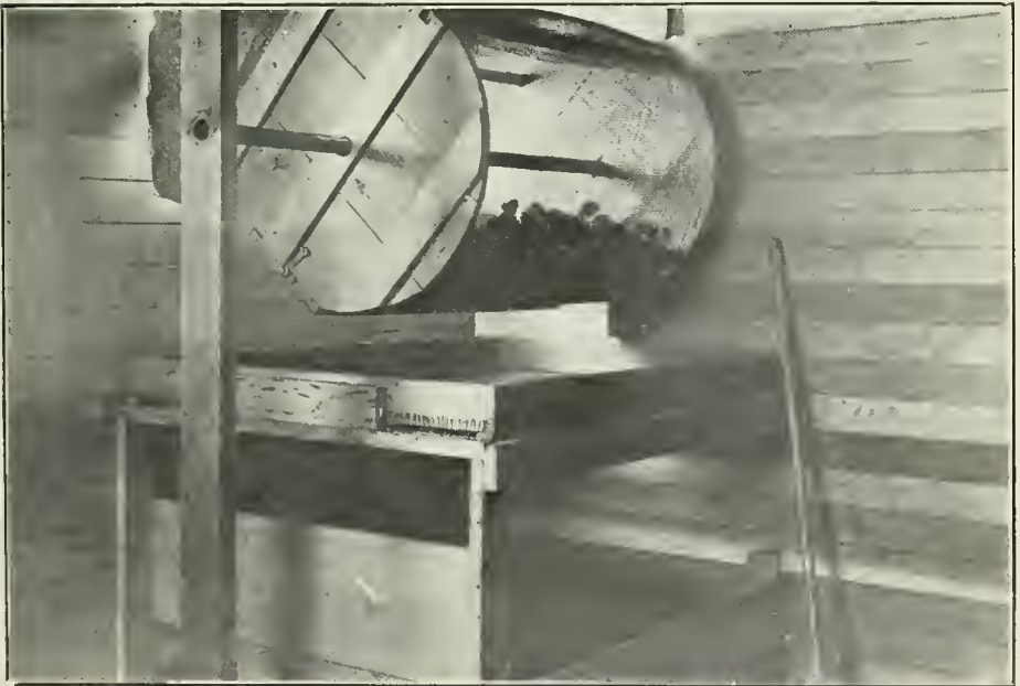
Cylindrical Screen for shaking out seed, Seedhouse at Forest Nursery Station, Indian Head, Sask.
