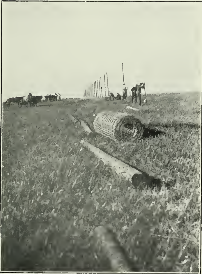
Erecting Fence around Buffalo Park.
