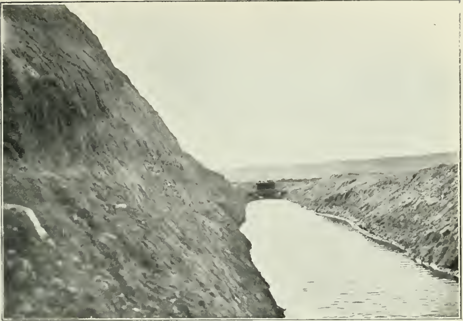
Thirty-five-foot cut for Ditch, East End, Sask.
