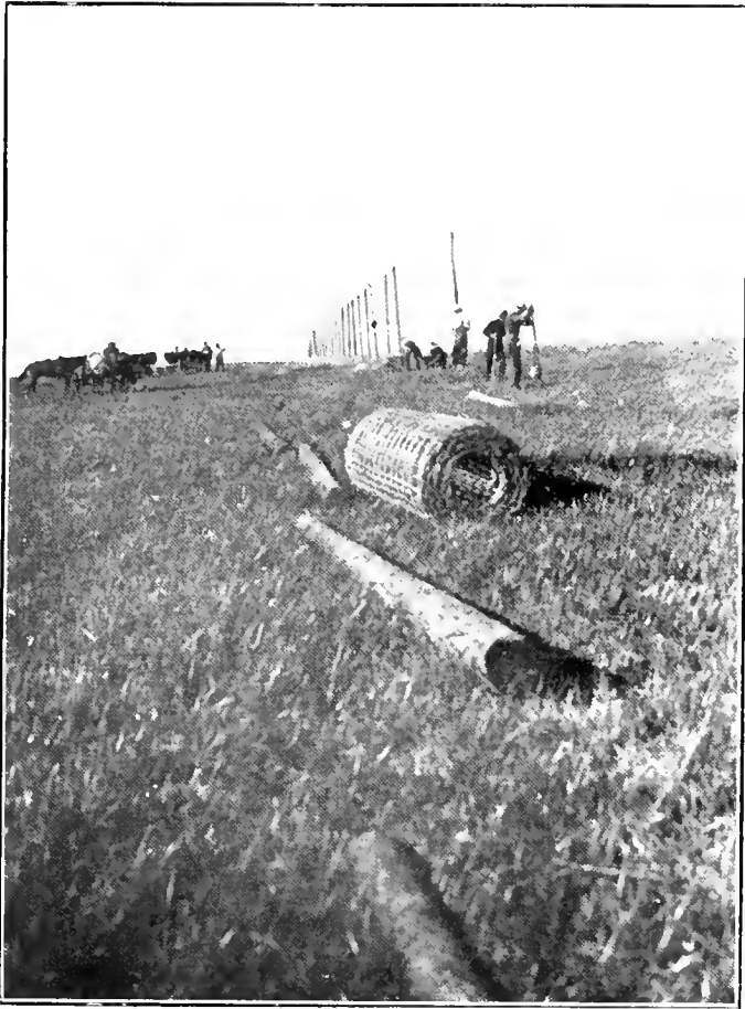
Erecting Fence around Buffalo Park.
