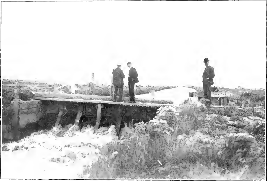
Head-gate on Irrigation Ditch, Alberta Railway and Irrigation Company's scheme.
