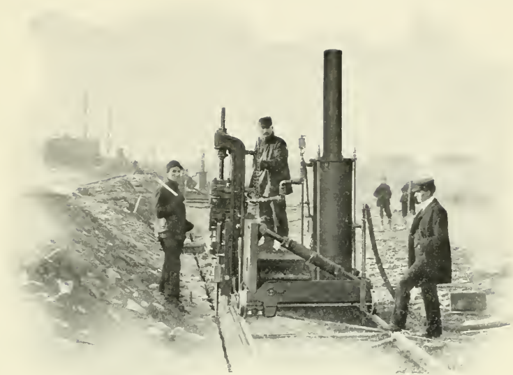
Channelling Machine at Work.
