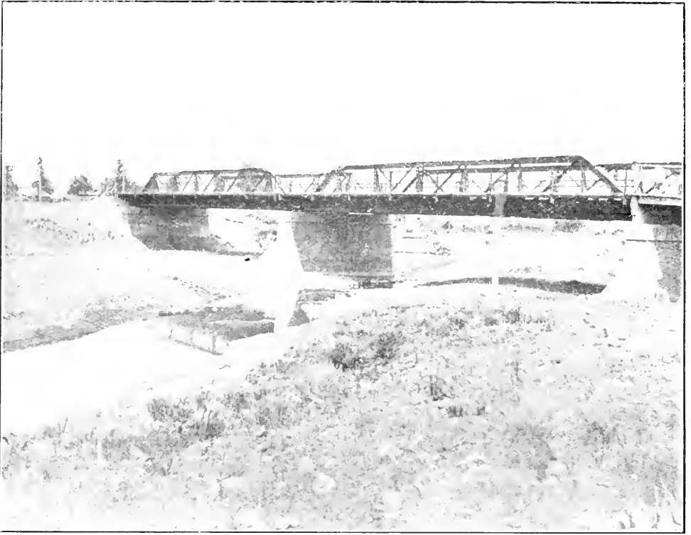
Traffic Bridge over Lee Creek at Cardston, Alta
