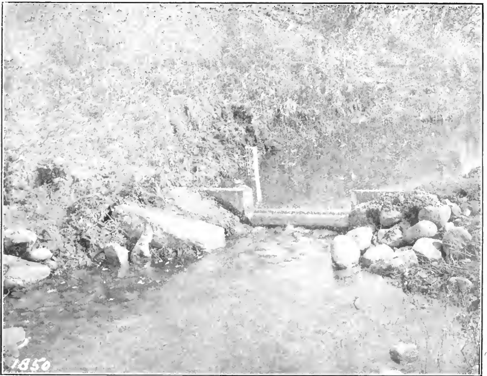
Sharp-crested, Rectangular, Wooden Weir.
