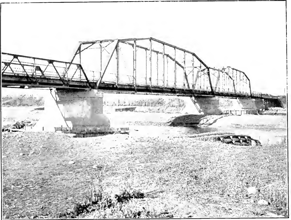
Traffic Bridge over Oldman River, near Macleod, Alta.
