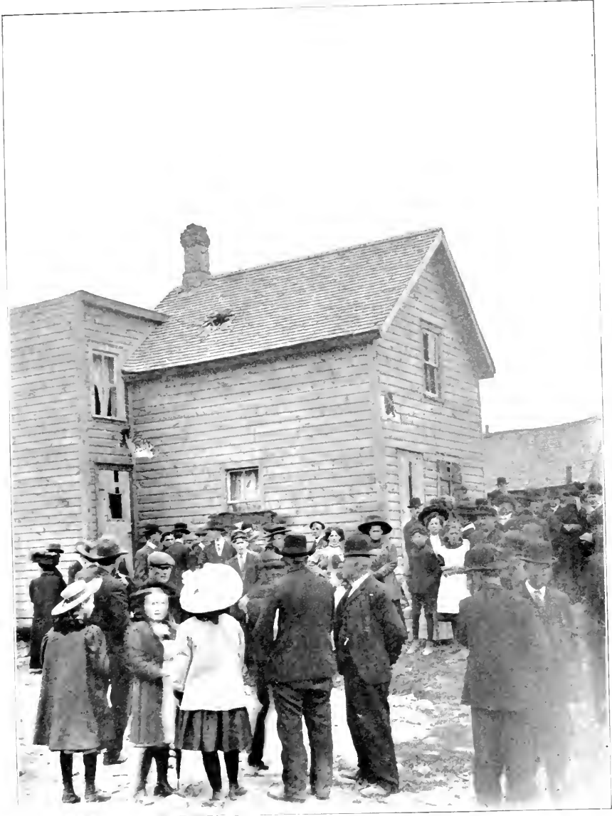
View showing where stone struck house and rebounded: killing one person and injuring another.
